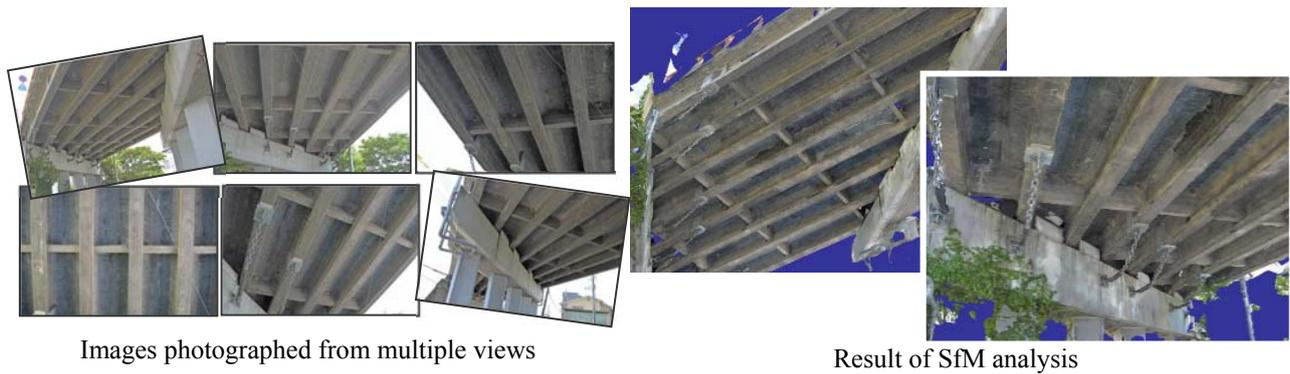
Fig. 4 Example of construction of 3D model by SfM
