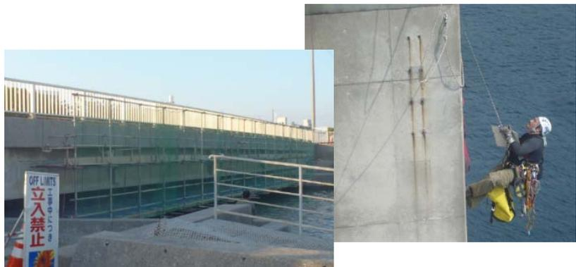
Fig. 1 Inspection of bridge pier by suspended scaffold and rope access
